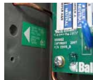
Ground in System Enclosure
