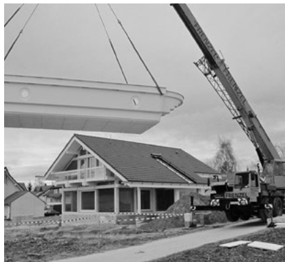
Insertion via crane
