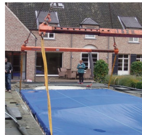
The pool is prefabricated in our factory, not on site. It is delivered to your location with a special transporter, either upright or on its base. Pools in segments are also possible - the flange is reworked on site with mosaic.
