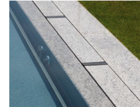
CONCEALED OVERFLOW CHANNEL
