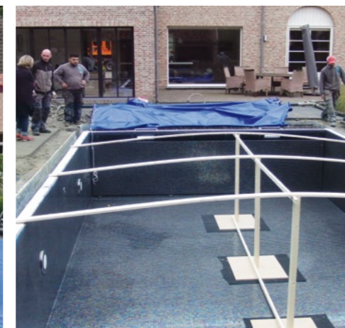
The pool is prefabricated in our factory, not on site. It is delivered to your location with a special transporter, either upright or on its base. Pools in segments are also possible - the flange is reworked on site with mosaic.
