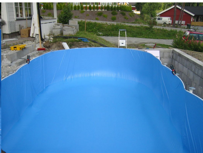
4. Bassengpose ferdig montert under vakuüm
