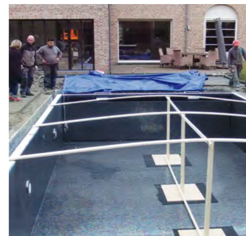
The pool is delivered to your location with a special transporter, either upright or on its base. Pools in segments are also possible - the flange is reworked on site with mosaic.
