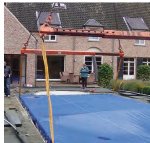
The pool is delivered to your location with a special transporter, either upright or on its base. Pools in segments are also possible - the flange is reworked on site with mosaic.
