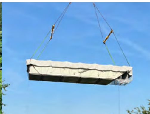
Installation of the MLine pool by crane.
