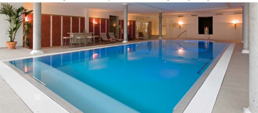
Hotel pool with overflow channel and gutter grating.
