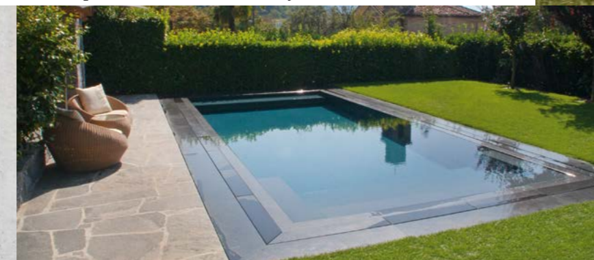
Outdoor pool with stone-covered overflow channel.
