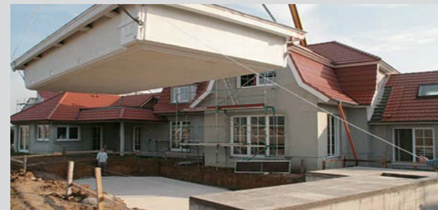
Concrete floor slab. Backfilling with lean concrete or modern insulating concrete.
