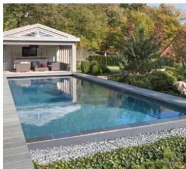
Overflow channel at the front side
