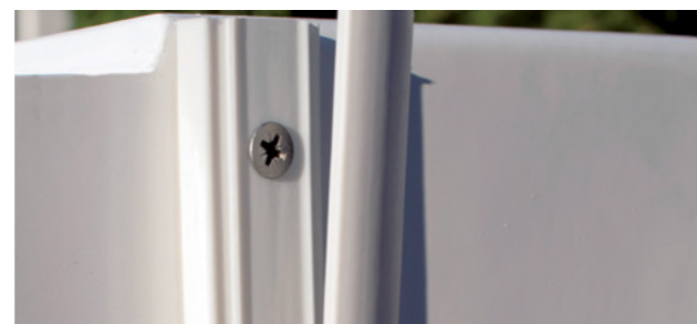
PVC liner can be fixed with a clamp plate or glued/ welded on a PVC strip.
