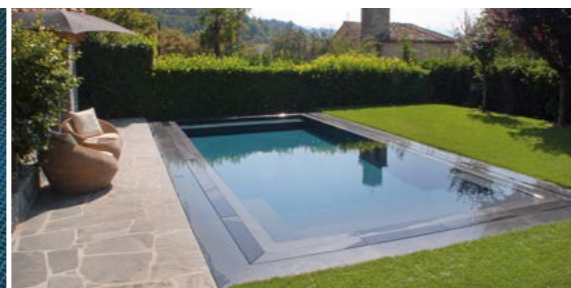
STONE COVERED OVERFLOW CHANNEL
