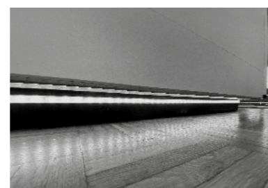
Lighting of the baseboards, LED white
