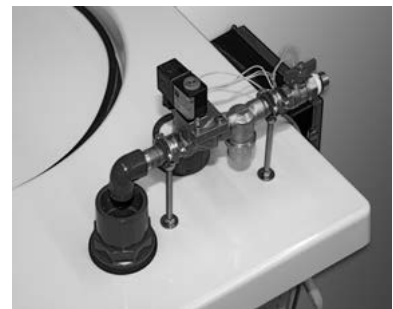
Water level and pump control, incl. mains water solenoid valve
